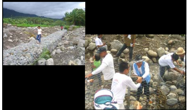
small-scale mitigation projects: gabions as flood mitigation measure
