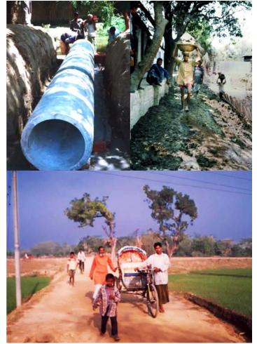
(top left) Laying drainage pipes, (top right) Using mud to raise road, (bottom) Finished raised and drained road
