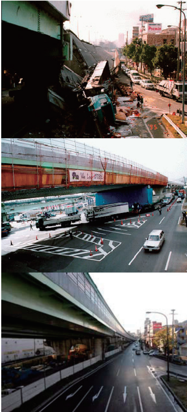
Highway in National Artery Road No.43 at Iwaya after the 1995 earthquake, 1996, and 2005.
