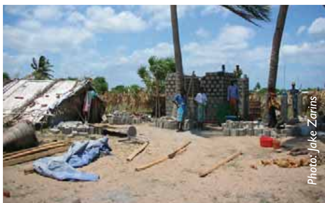
Core shelter under construction
