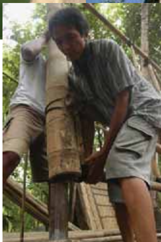
Connecting a vertical post to the foundation
