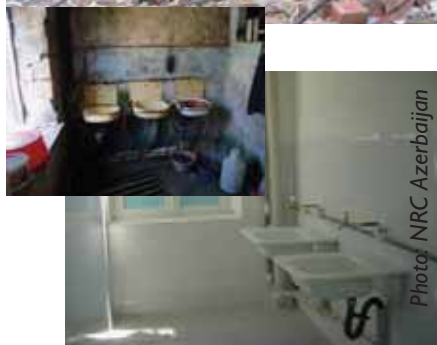
Bathrooms before and after upgrade
