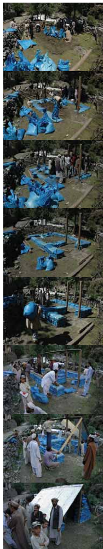
Building one of the transitional shelters
