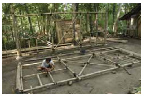
Prefabrication of a wall panel
