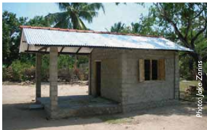
Completed core shelter
