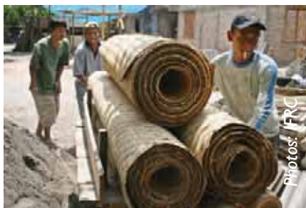
Transporting bamboo mats to a construction site
