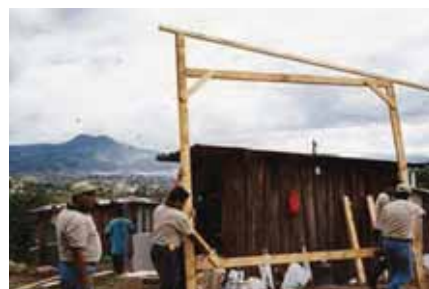
Shelter assembly using prefabricated walls
