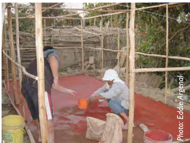
Making the concrete floor slab
