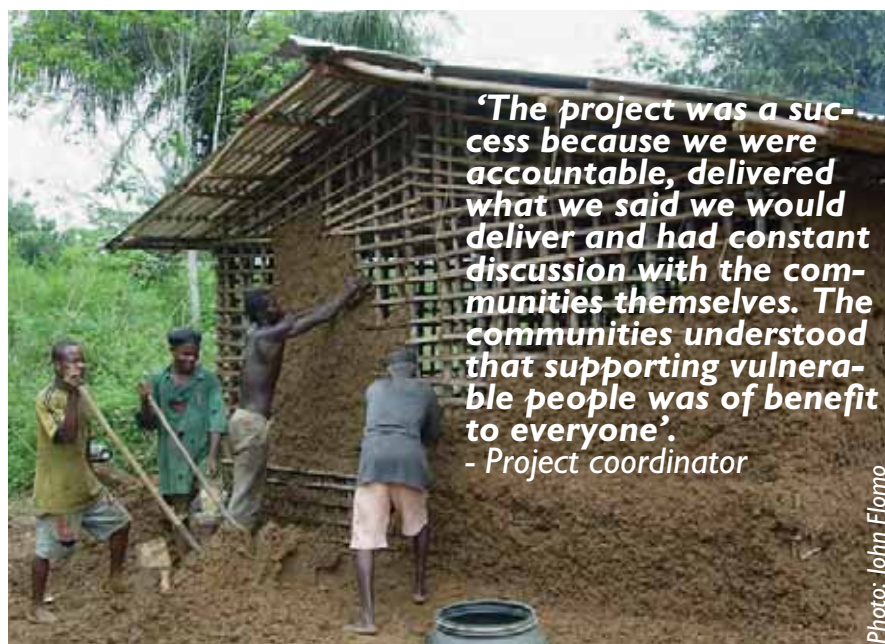
Traditional shelters under construction
