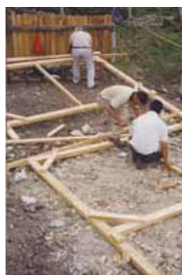
Prefabricating walls
