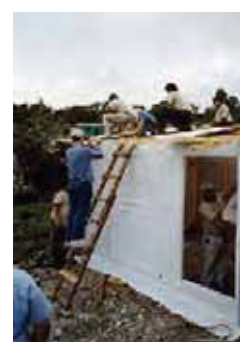
Covering the roof with corrugated iron
