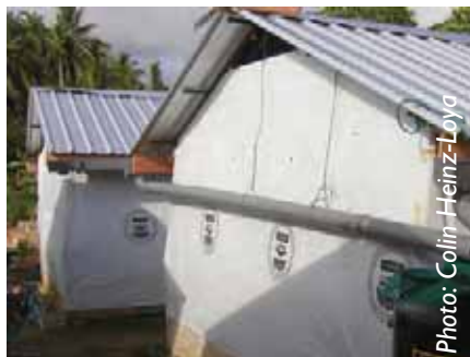
Shelters built with tanks for rainwater harvesting
