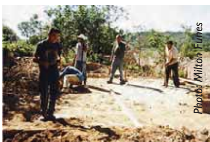
Marking out the site for a shelter
