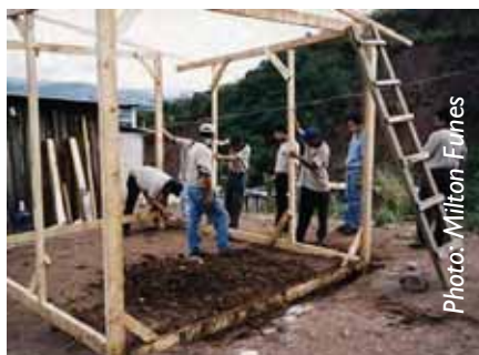
Completing the frame
