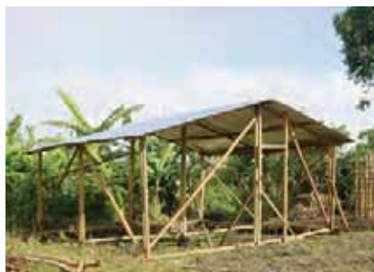
Structural skeleton of a house, showing cross-bracing
