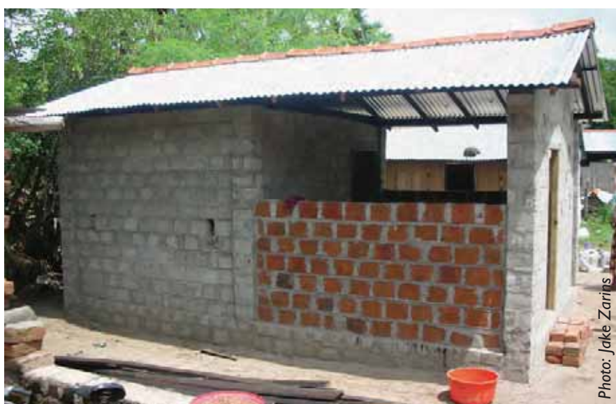
A durable upgrade of a core shelter
