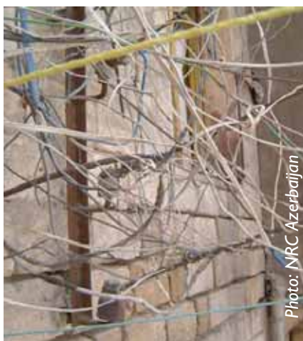
Wiring before upgrade
