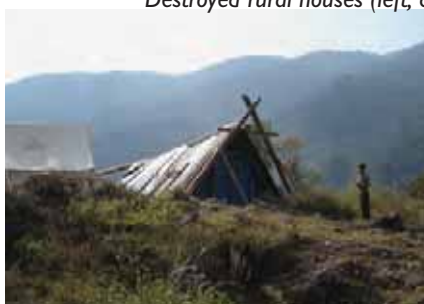
Self-built shelters in Kashmir built using reclaimed materials only ten days after the earthquake
