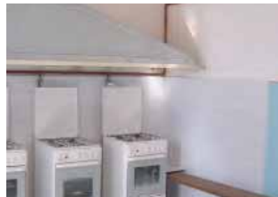
Kitchens before and after upgrade
