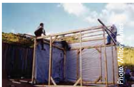
Covering the frame
