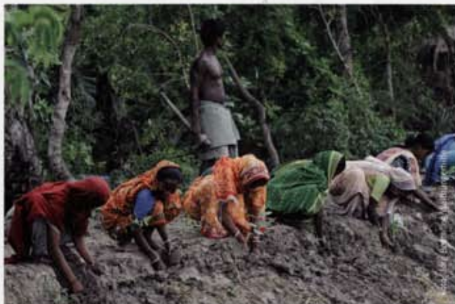
India: Dike protection
