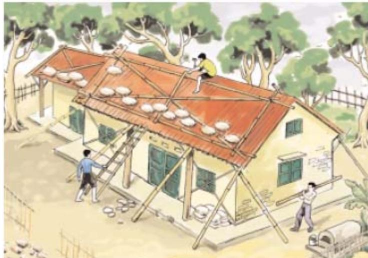
**Picture 17 Reinforcing houses before typhoons**
