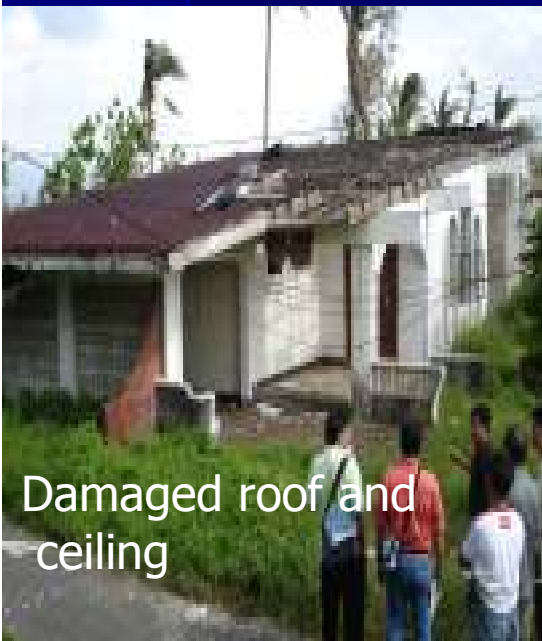
Damaged ceiling framing, eaves, fascia; broken window glazing;
