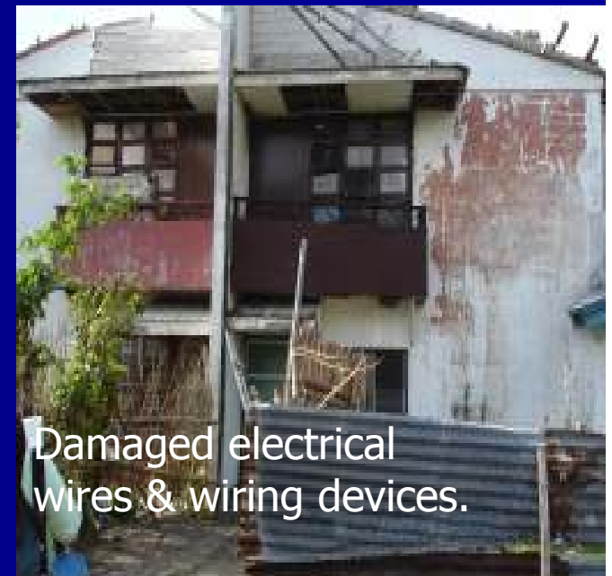
Damaged ceiling framing, eaves, fascia; broken window glazing;
