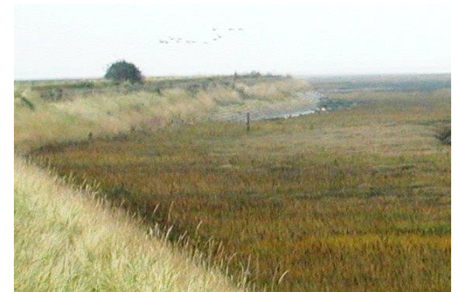
Figure 2 Saltmarsh fronting sea defences at Tillingham, Dengie Peninsula, UK southern North Sea coast. Note earthen bank in front of wide saltmarsh (foreground) and the need for a re-inforced sea defence (background left) where coastal erosion has resulted in a narrow saltmarsh with fronting mudflat (photo: I Moller)
