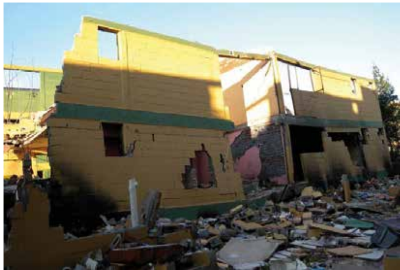
Image 2: A building with a collapsed ground floor as a result of the February 2010 earthquake in Chile. Source: Brzev, Astroza and Yadlin, 2010 22 .
