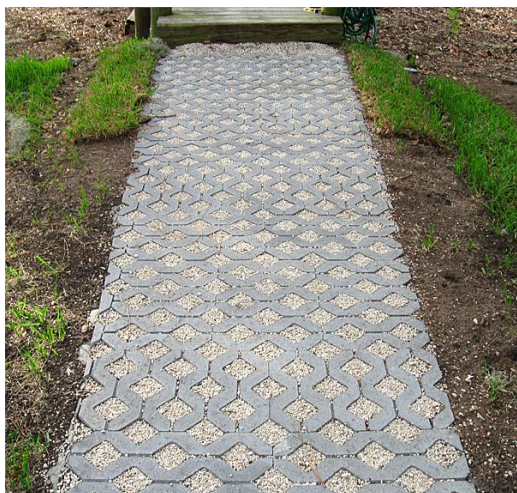
Figure 5: Installed Permeable Pavers
