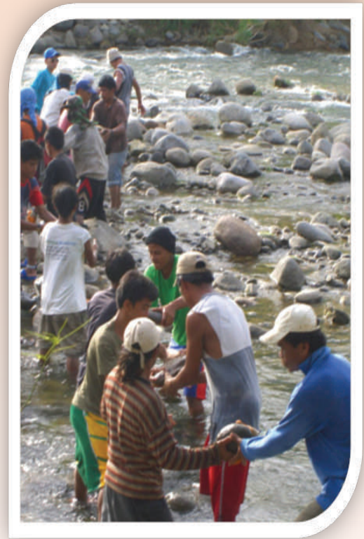
Above: Gabion wall construction as flood mitigation measure.
