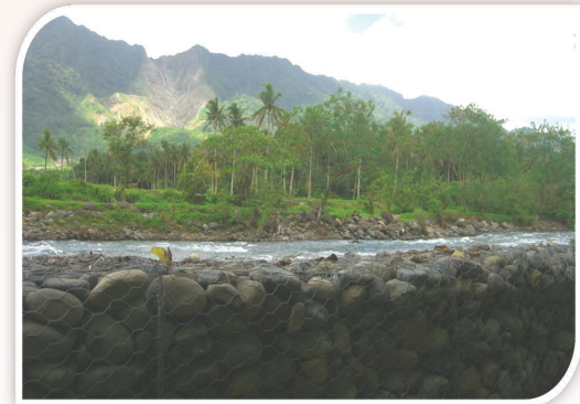
Below: Already constructed gabion wall
