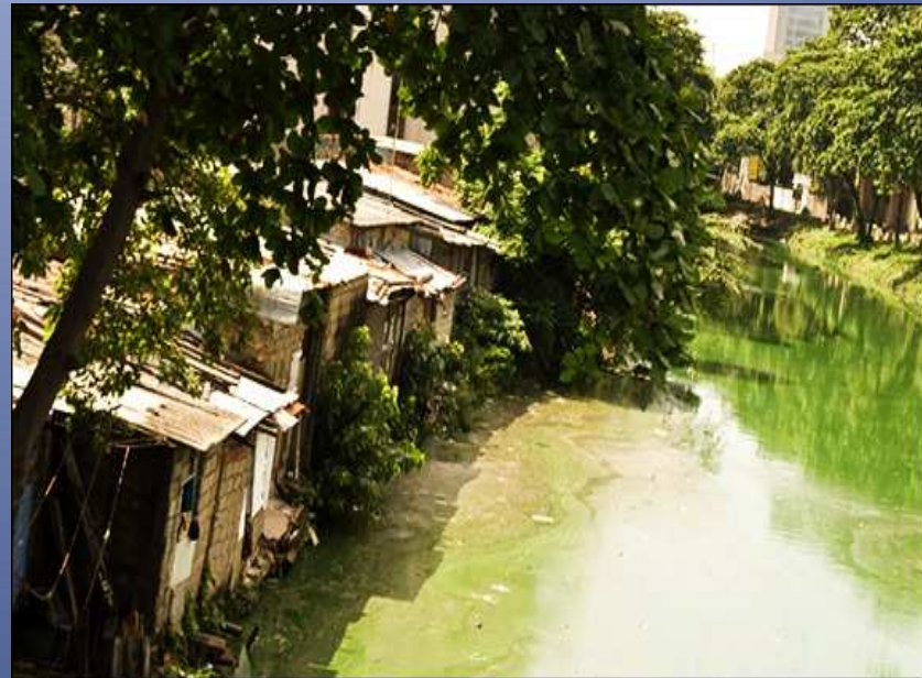
Unauthorised structures on a canal reservation
