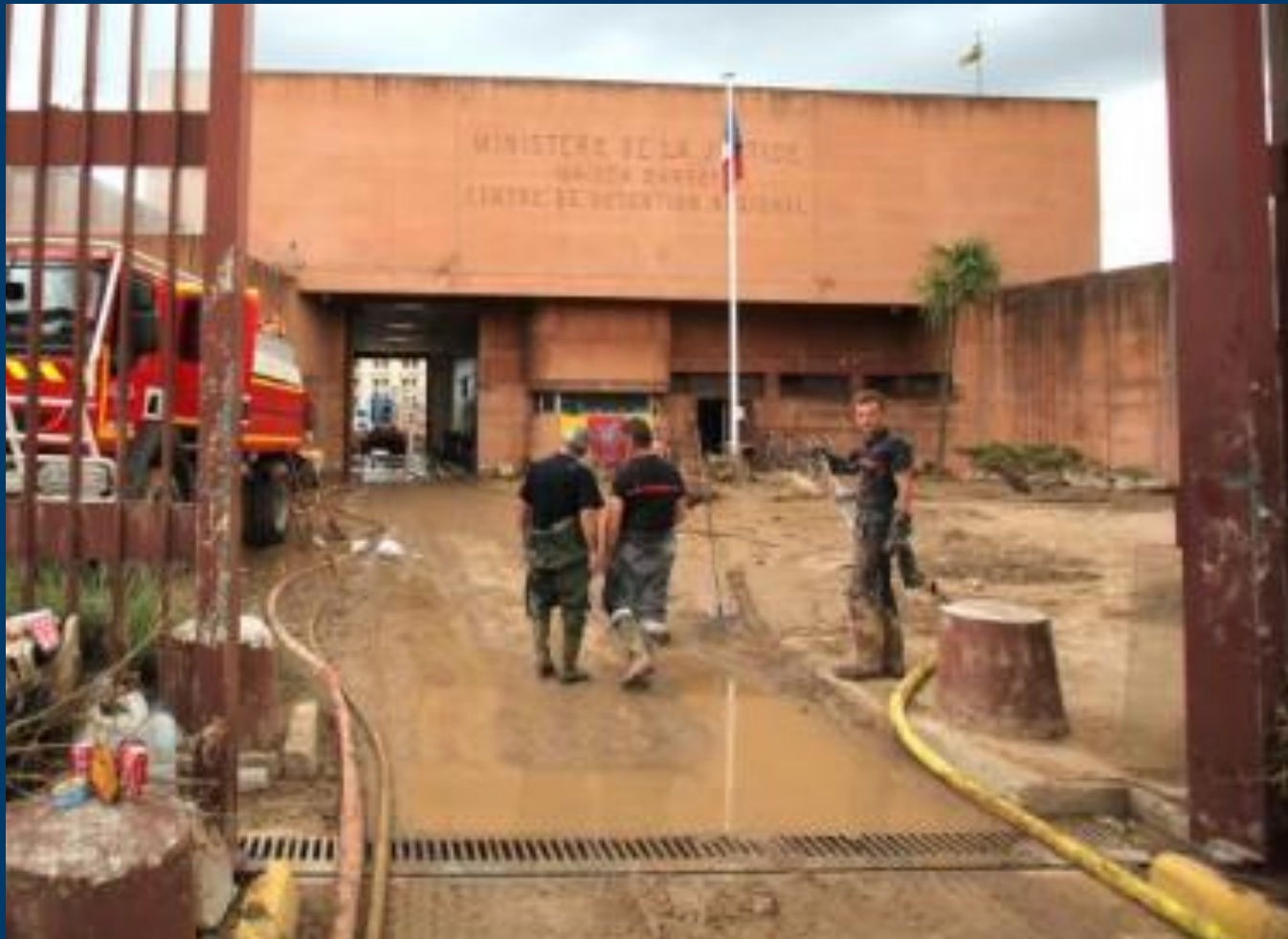
Damage to the Draguignan prison, France, in June 2010 ( Anonymous )
