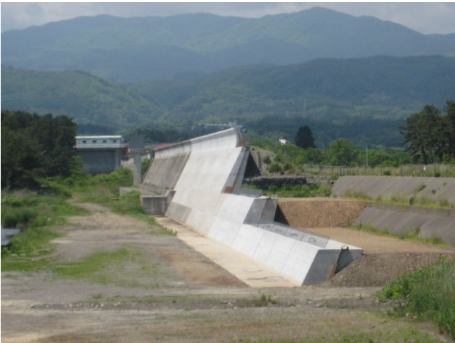
Photo3-2-3 Tsunami embankment being built in Noda village
