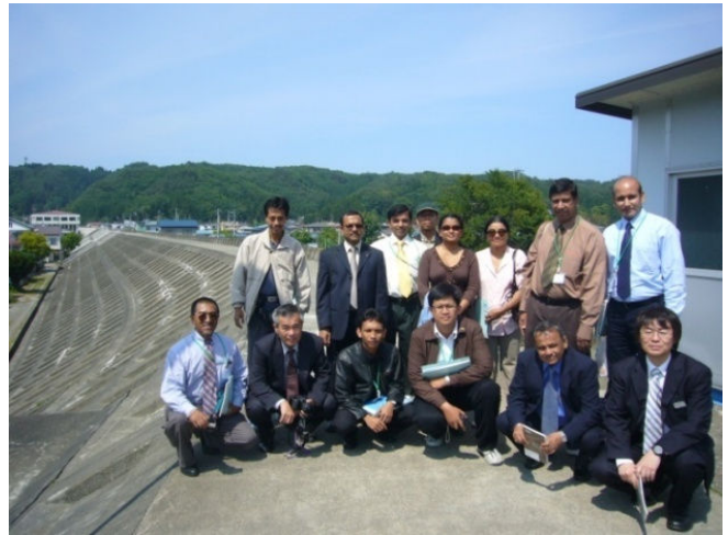
Photo3-2-8 On the Taro sea wall
