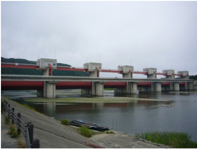
Photo3-2-7 Water gate at the mouth of the Omoto River
