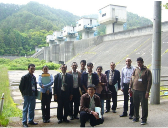
Photo3-2-1 Tsunami Watertgate in Fudai village
