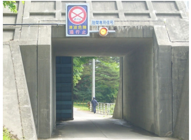
Photo3-2-2 Demonstration of the gate closing
