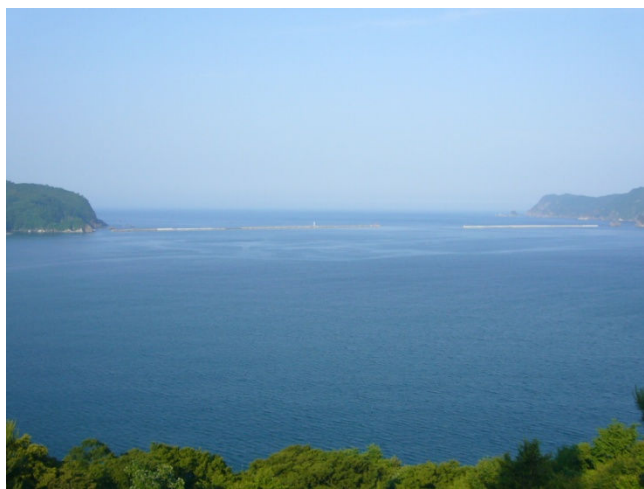
Photo3-2-9 Tsunami breakwaters in Kamaishi
