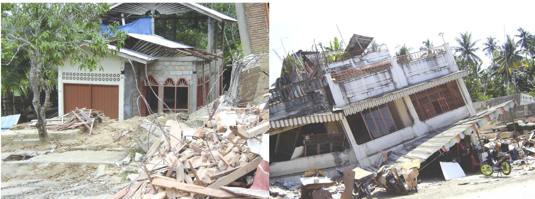
Pictures 4 and 5 Damage caused by earthquake at Nias Island.
