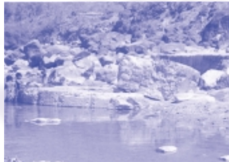
Figure 2 Huge slumping and bridge collapse after heavy rainfall (Butwal-Nepalganj Road, West Nepa) Source: Deoja, et.al 1991
