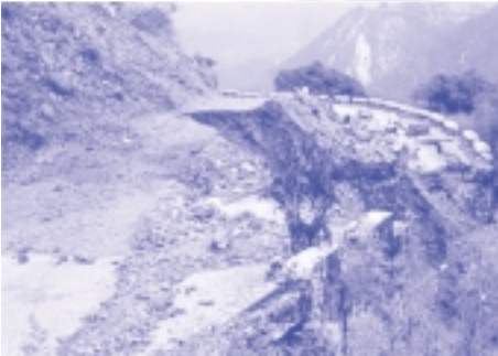
Figure 3, Slope failure from earthquake and heavy rainfall in 1998 (Dharan-Dhankuta Road, Nepal) Source: Deoja, et.al 1991
