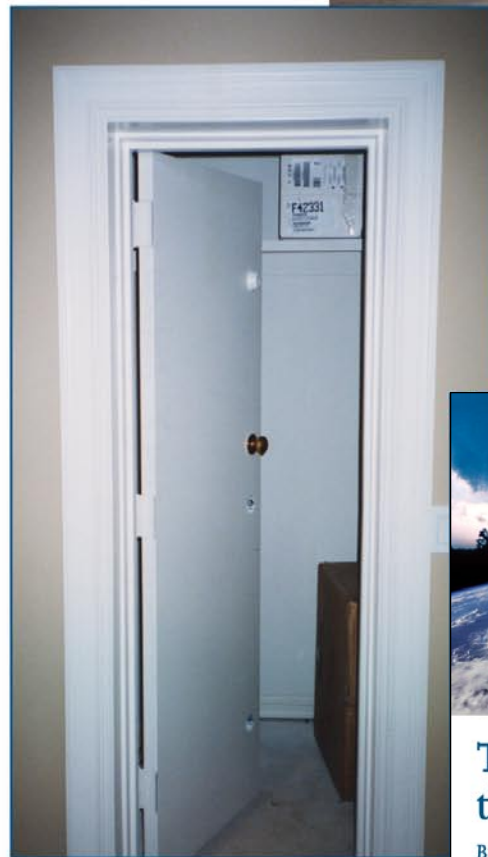
Views of residential safe room construction. Completed safe room, left, functions as a closet during daily use. Doors must meet FEMA 320 or National Performance Criteria for Tornado Shelters standards.
