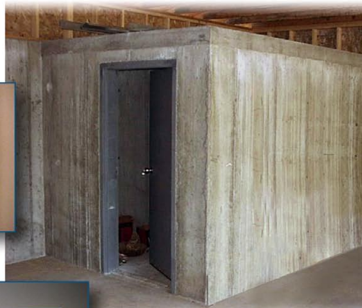
Views of residential safe room construction. Completed safe room, left, functions as a closet during daily use. Doors must meet FEMA 320 or National Performance Criteria for Tornado Shelters standards.
