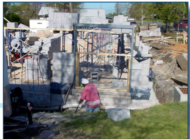
Construction of a College Station elementary school shelter. (SOURCE: WAPDD)
