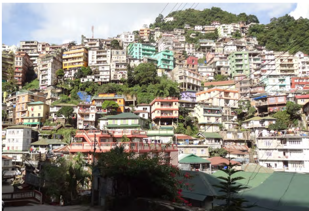
Figure 9. Vulnerable buildings on a steep slope where a collapse would endanger buildings below (Photo credit: Janise Rodgers, GHI)
