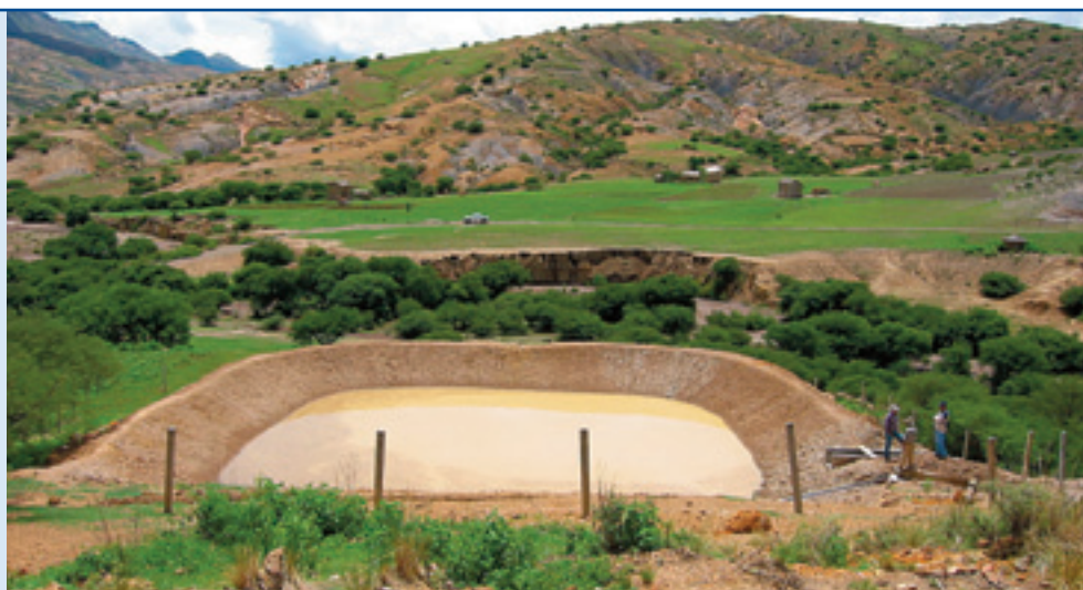
Figure 9: Rainwater harvesting basin for complementary irrigation
