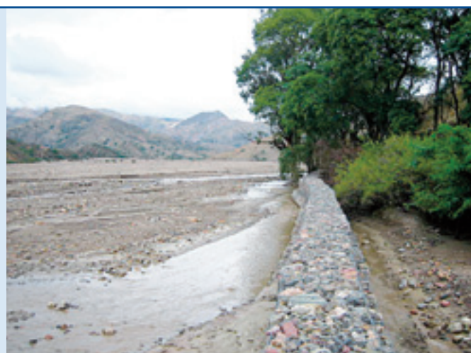
Figure 11: Protecting the riverbank slope on which San Pedro de Buena Vista is located
