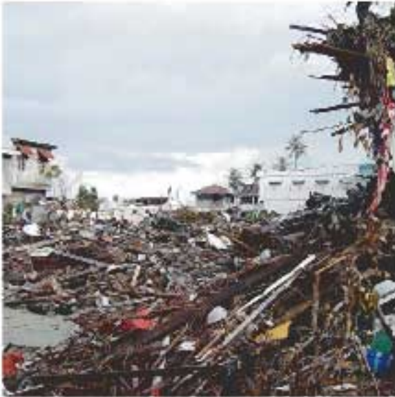
Homes and Shops Turned to Rubble
