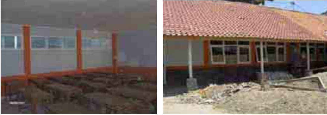
Figure 87: Various stages of the retrofitting process
