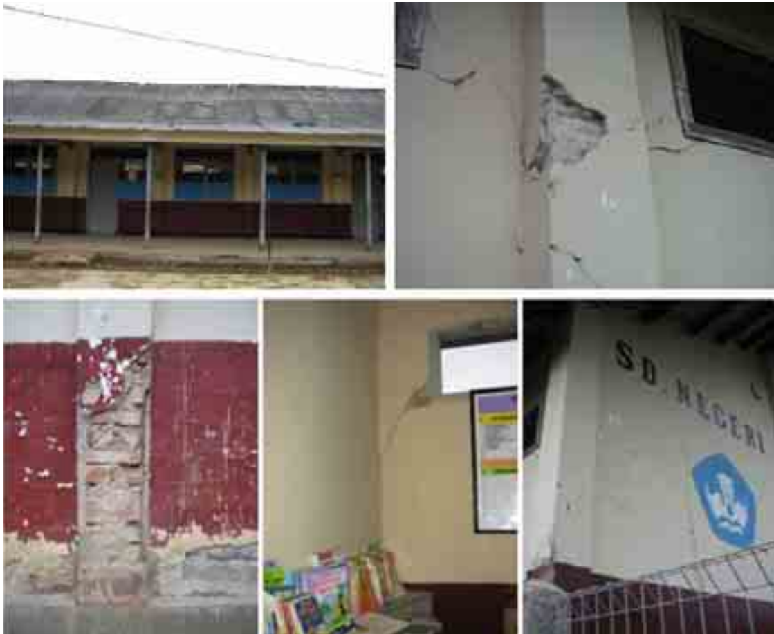
Figure 83: Existing condition of SD Padasuka II
