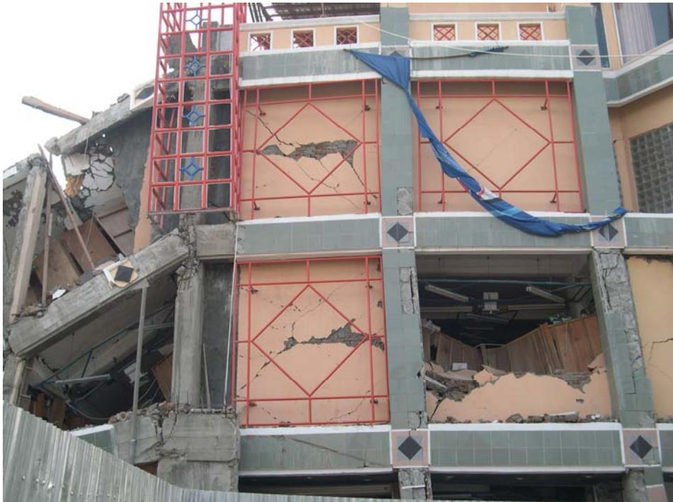
Photograph 2- Reinforced concrete building, Banda Aceh. An example of poor beam-column joints. Refer Recommendation Nos. 10 & 19.
