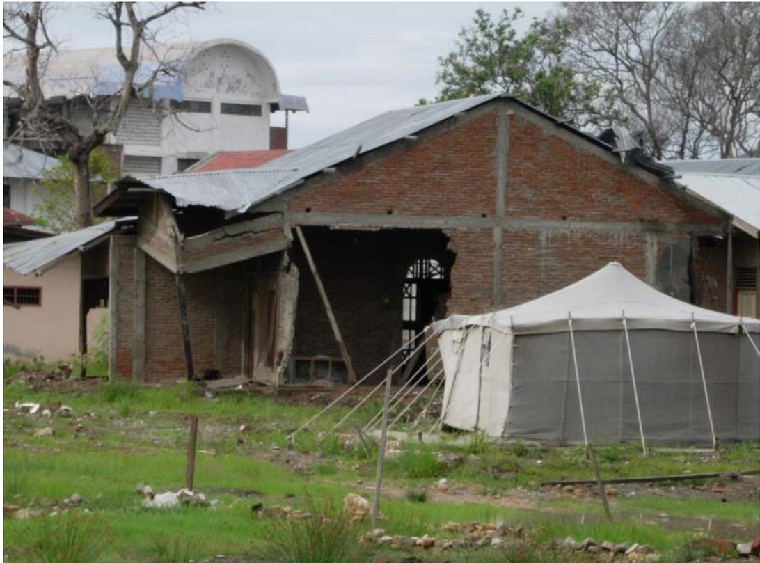
Photograph 3- Confined brick masonry building, Banda Aceh. When walls collapsed practical columns were overloaded. Refer Recommendation Nos. 15 & 18.
