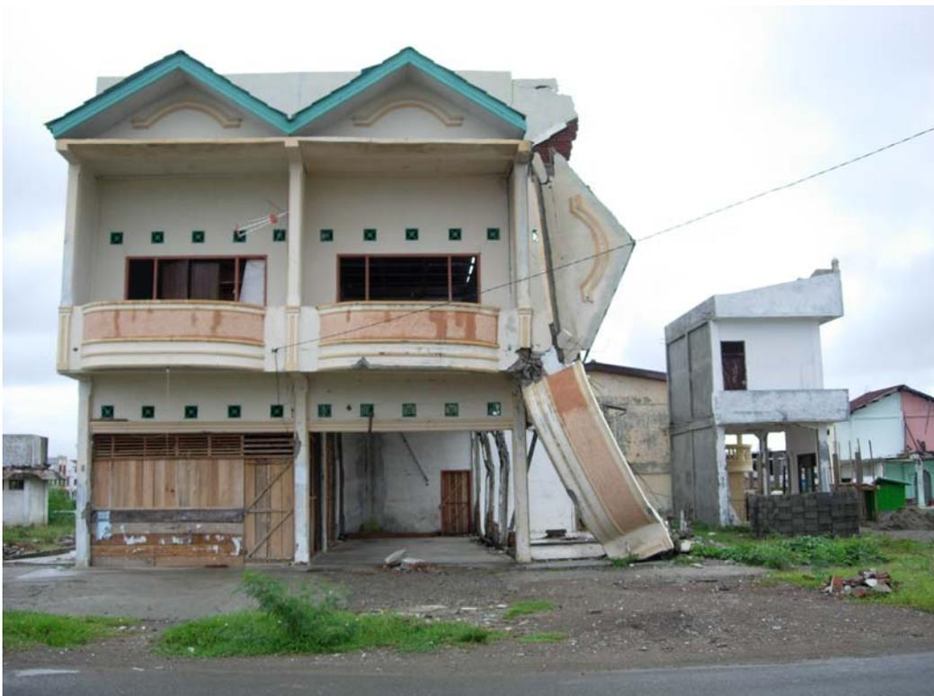
Photograph 6- Typical Building, Banda Aceh. Failure of heavy architectural elements.
