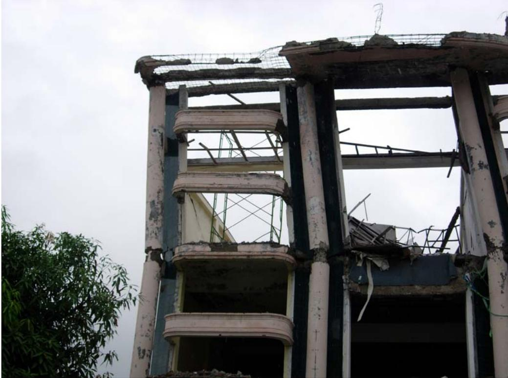
Photograph 5- Reinforced concrete Hotel, Banda Aceh. Failure of beam column joints.
