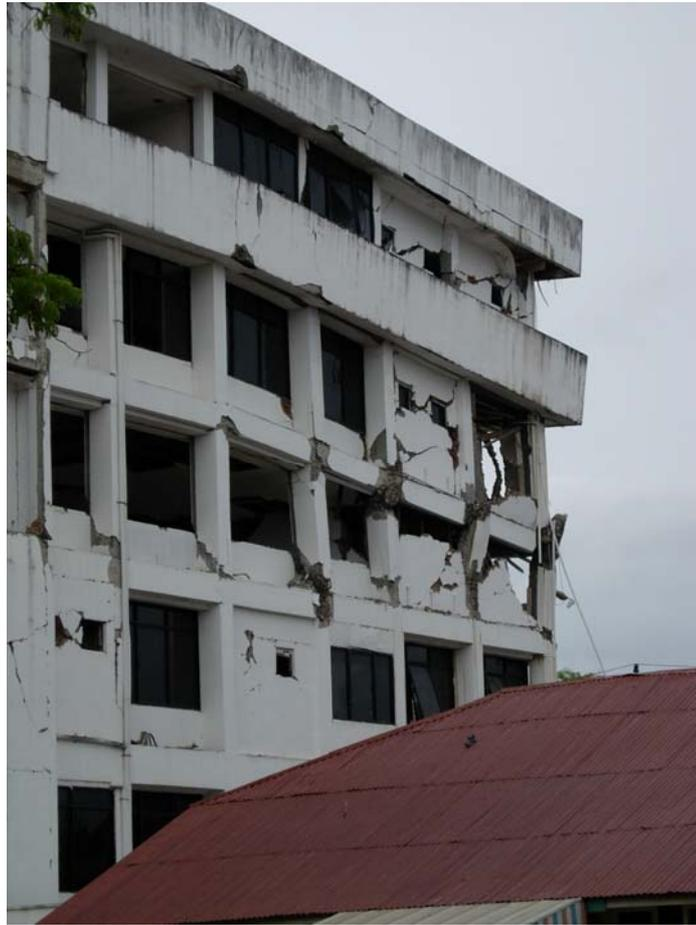
Photograph 7- Reinforced concrete moment resisting frame building, Banda Aceh.
