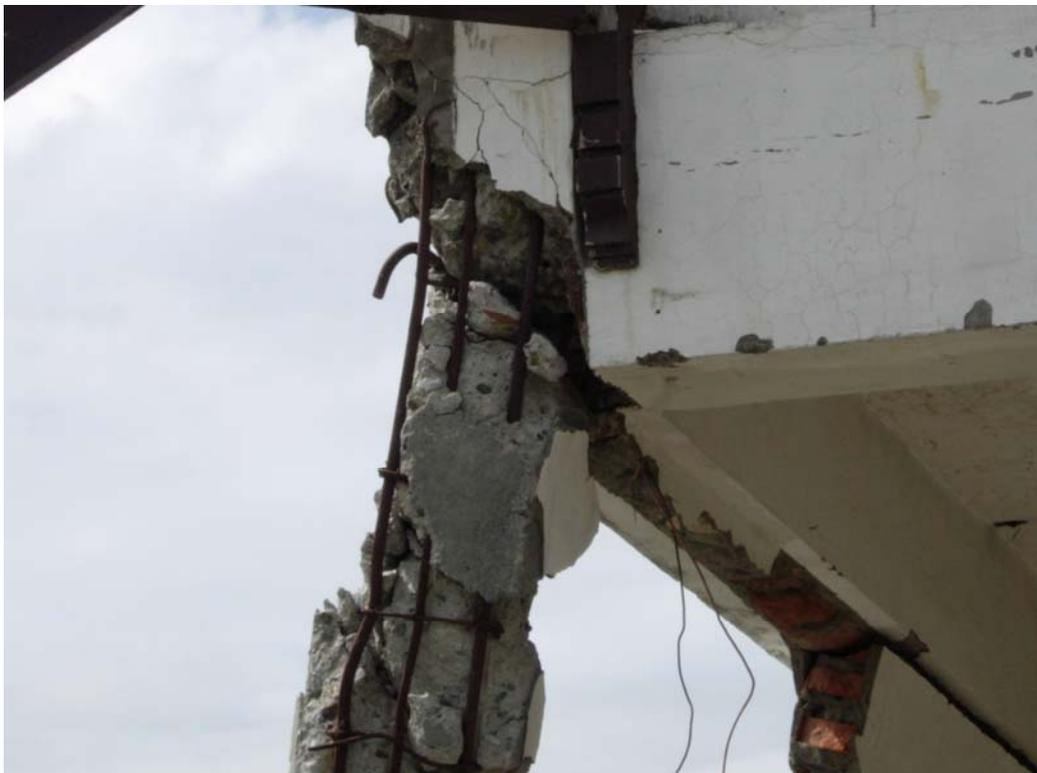
Photograph 4- Reinforced concrete building, Banda Aceh. Ties are too small and too widely spaced. Column has failed. Refer Recommendation No. 19.
