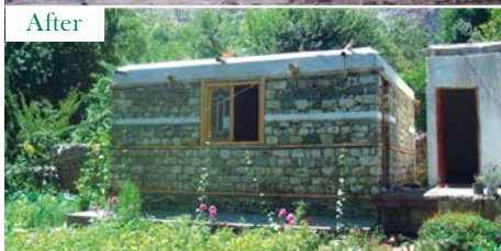
HRMP Reconstruction Project: Reconstructed house of Mr. Hazarat Shah, Gich, Ghizar, Northern Areas, Pakistan, 2008
