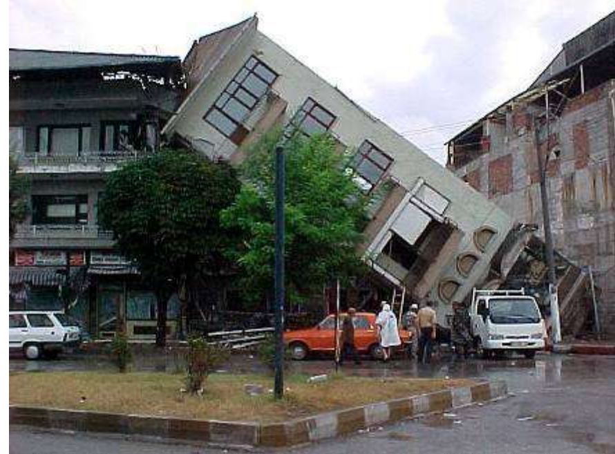
learning from earthquakes - Liquefaction
