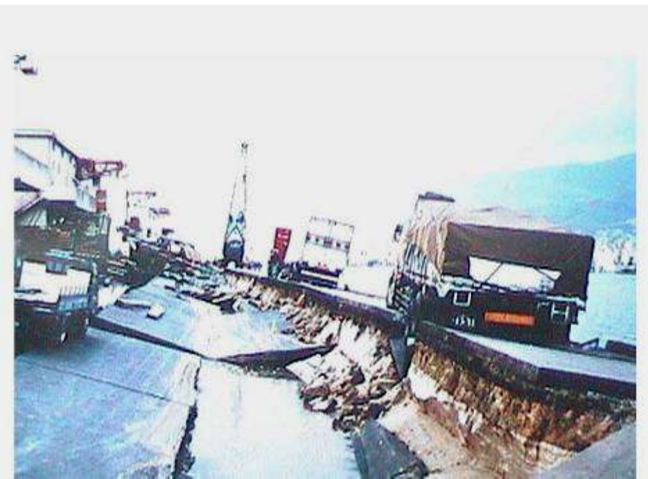
learning from earthquakes - Liquefaction
