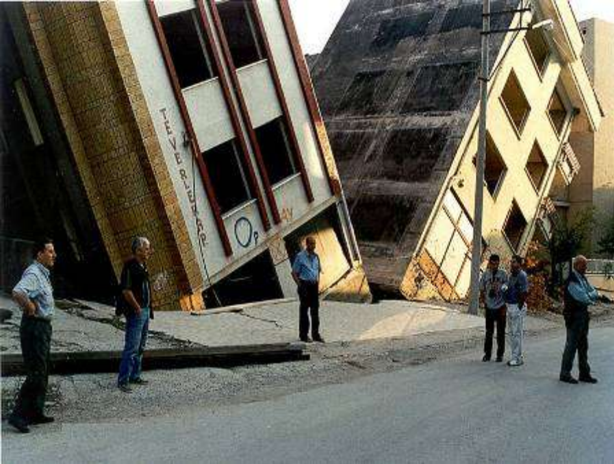
learning from earthquakes - Liquefaction
