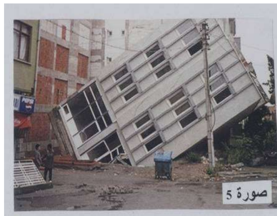
learning from earthquakes - Liquefaction
