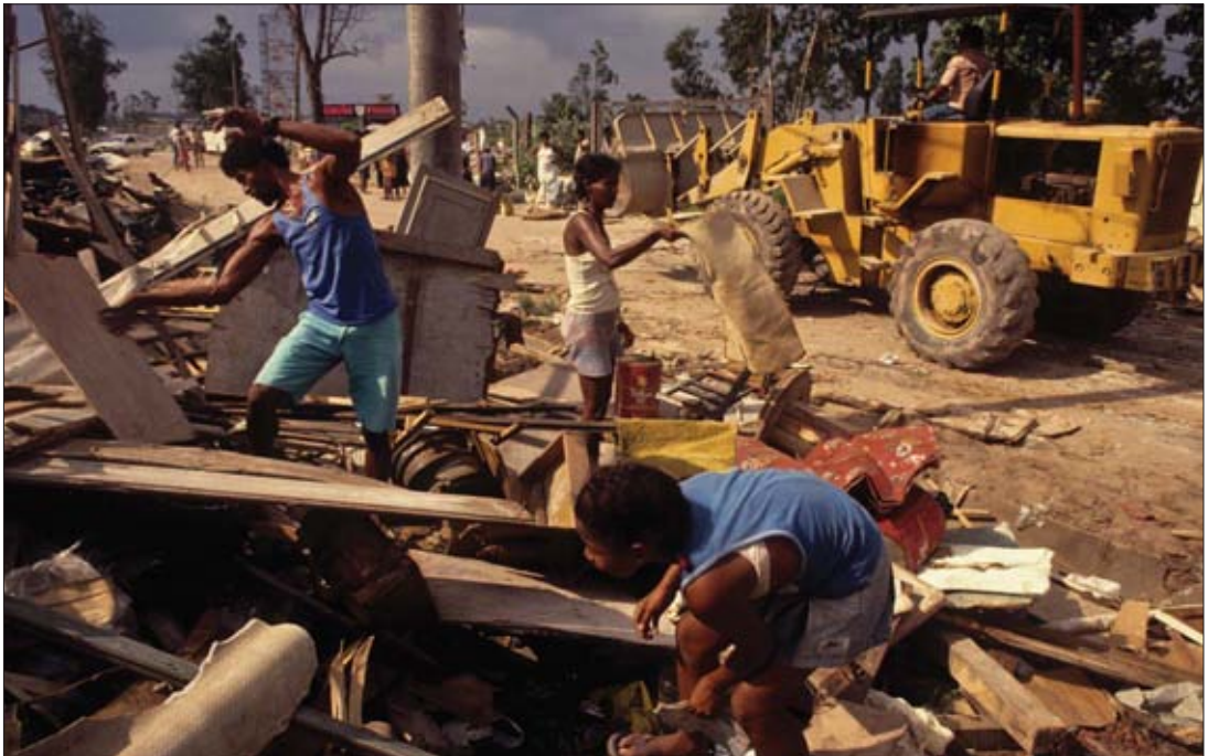
Forced demolition of slums is widespread in many countries
