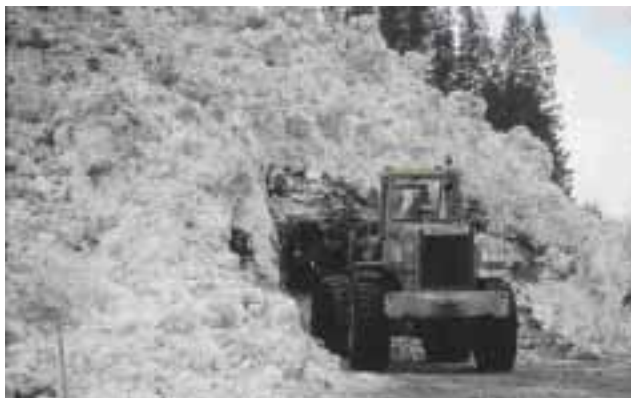
Figure 8.5: Large amounts of wet snow may pile up in flat areas when the front stops and additional volume from the tail of the avalanche accumulates on top of the snow that has come to rest (photo: NGI).
