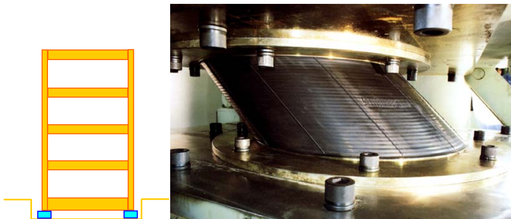
Figure 17. Base Isolation for Retrofitting
