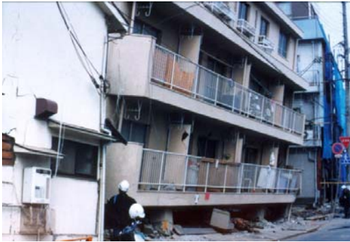
Figure 10. Damage of soft first-story buildings with construction age
