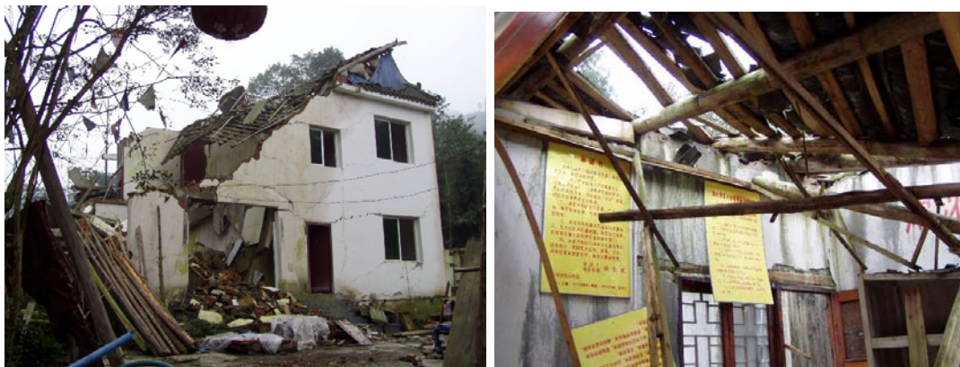
Figure 1. Un-reinforced brick masonry houses in Hongkou, Dujiangyan, Chengdu City, Sichuan Province, China
