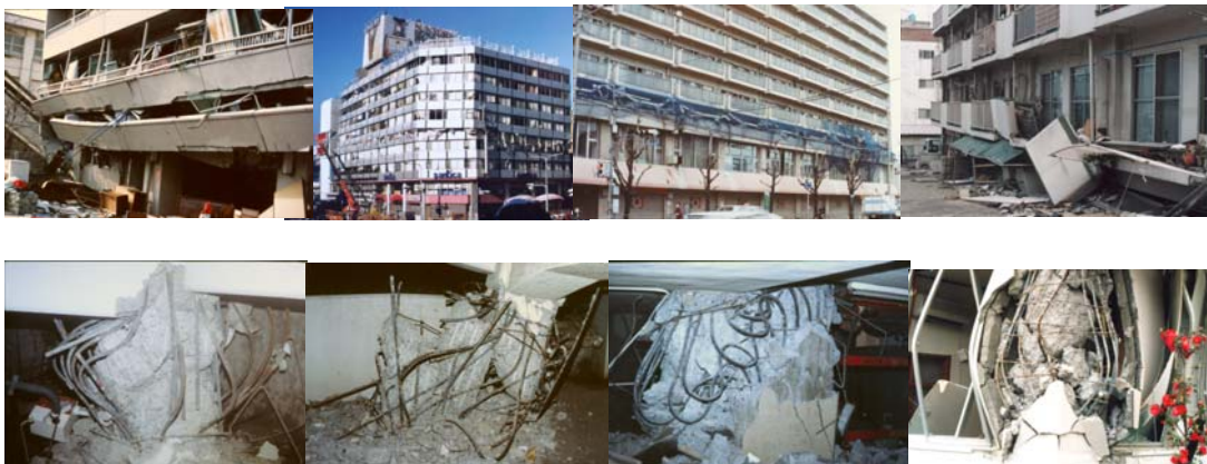
Figure 8. Reinforced concrete buildings in the 1995 Kobe disaster
