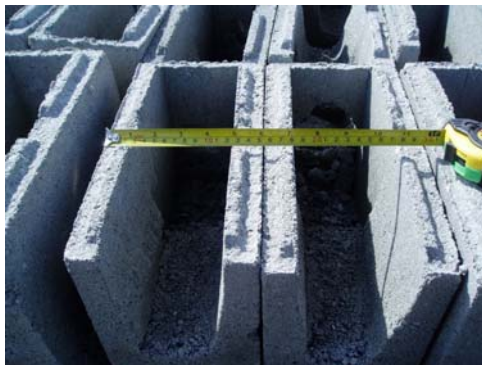
Figure 8. Interlocking masonry walls, poor quality blocks and no precision (Aceh)
