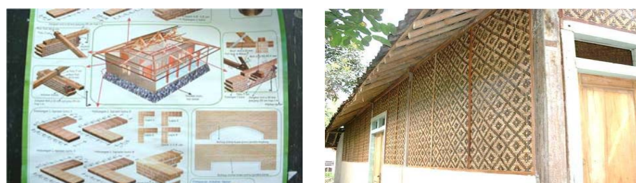
Figure 7. Poster for public awareness on earthquake resistant methods for non-engineered houses (Left) and Reconstructed (Temporary) House using local materials (Right), Java, Indonesia, September 2006
