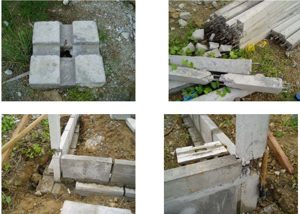
Figure 6. Walls using extra large size blocks with poor connections
