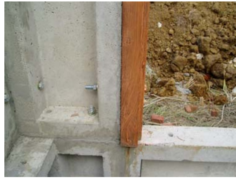
Figure 7. Pre-cast construction using 2 bolts for connections between components
