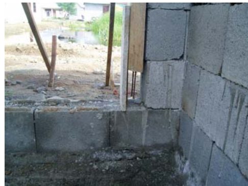
Figure 8. Interlocking masonry walls, poor quality blocks and no precision (Aceh)
