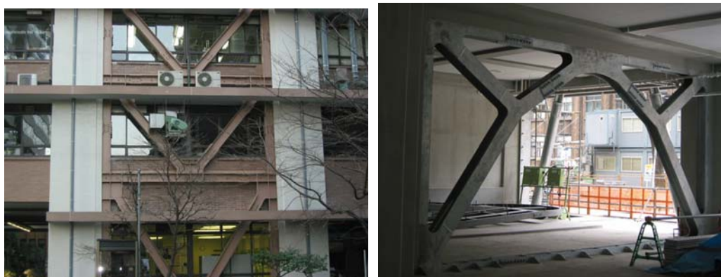
Figure 15. Detailing of wall-frame connection (Left) and Reinforcement of Columns (Right)
